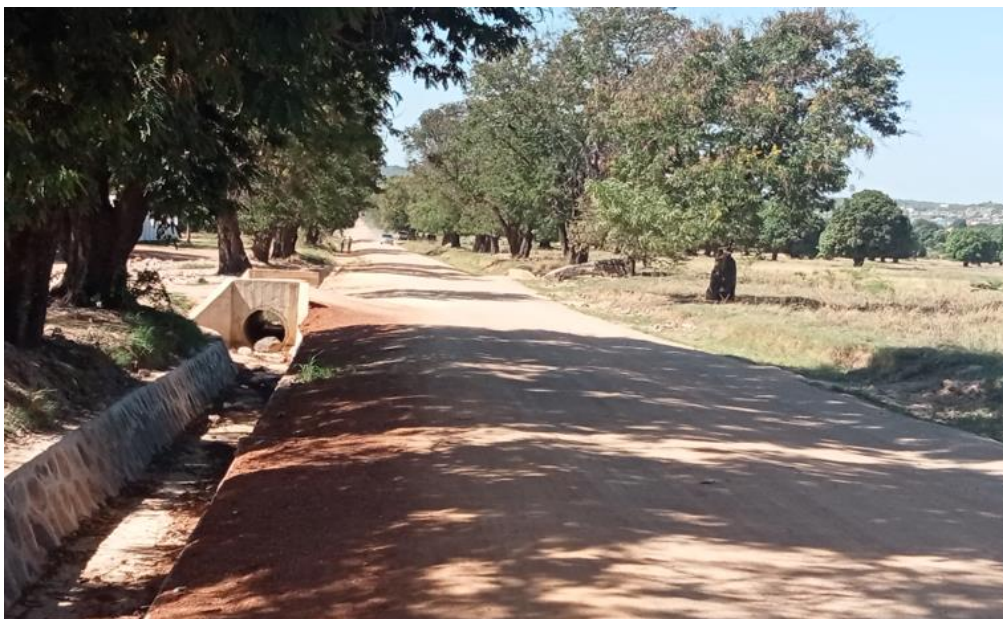
Figure 6.8: Culvert and drainage structure along Swetu road (Source: Fieldwork December 2021)
