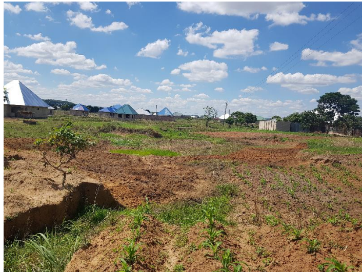
Figure 6.12: borrow pits left after soil taken for brick making in Kisarika IV(Nguzo Tanesco) road
