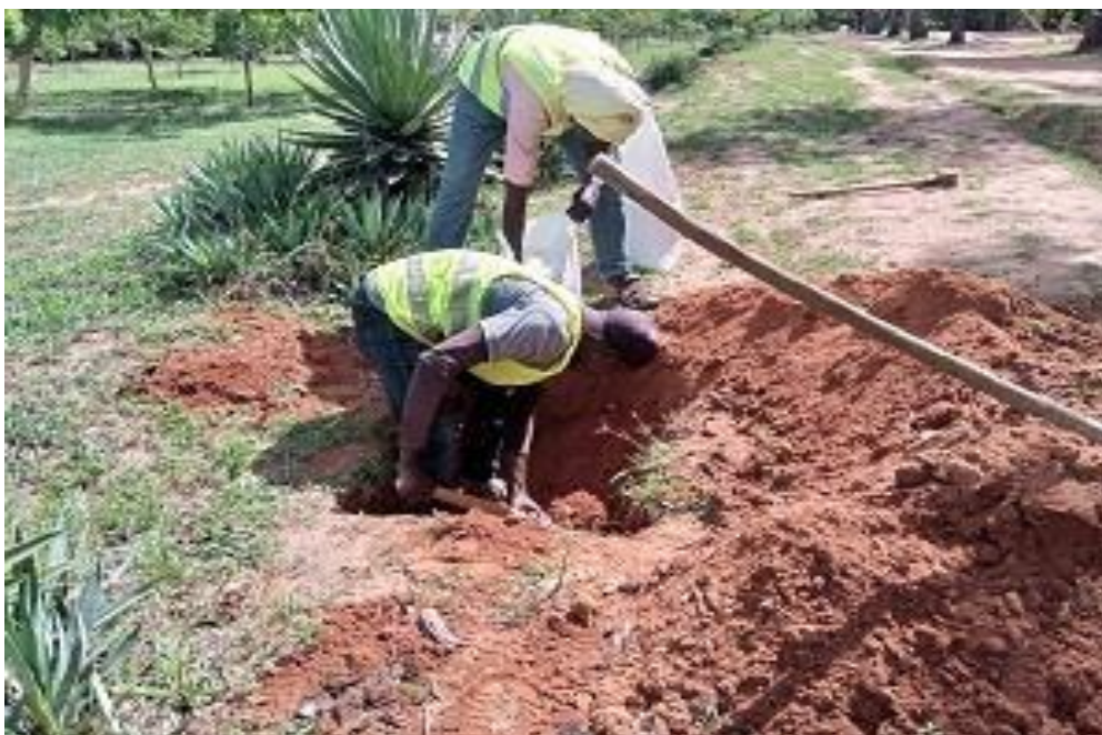
Figure 7; Test Pit excavated at km 1+750(Swetu road)
