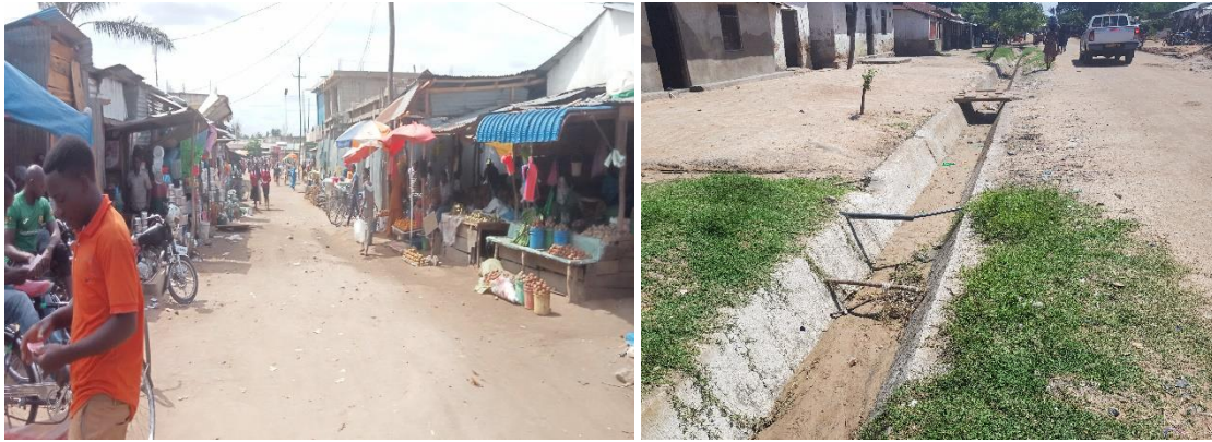
Figure 6.16: Public facilities to the Kanyenye I sub-project road (350m section) and Kanyenye III road
