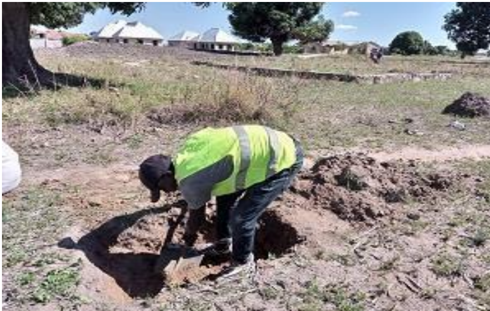
Figure 8: Test pit excavated at km 0+750(Kisarika road)
