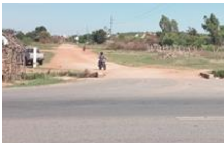
The starting point of the project road (Tabora-Nzega road)
