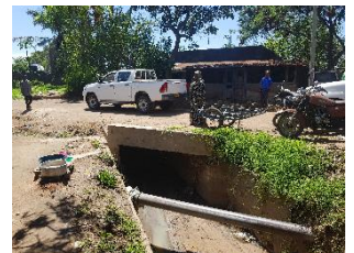
Existing drainage channels, electric power lines and water pipes along the Kanyenye II road
