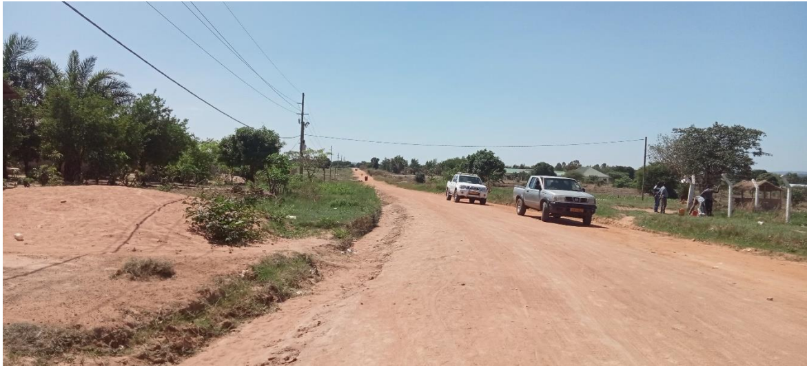
Figure 6.2: Powerlines parallel to the Maili Tano sub-project road
