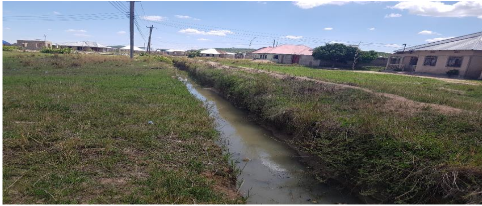
Figure 6.12: an existing drainage channel along the proposed Kisarika IV road (Source: Fieldwork, December 2022)
