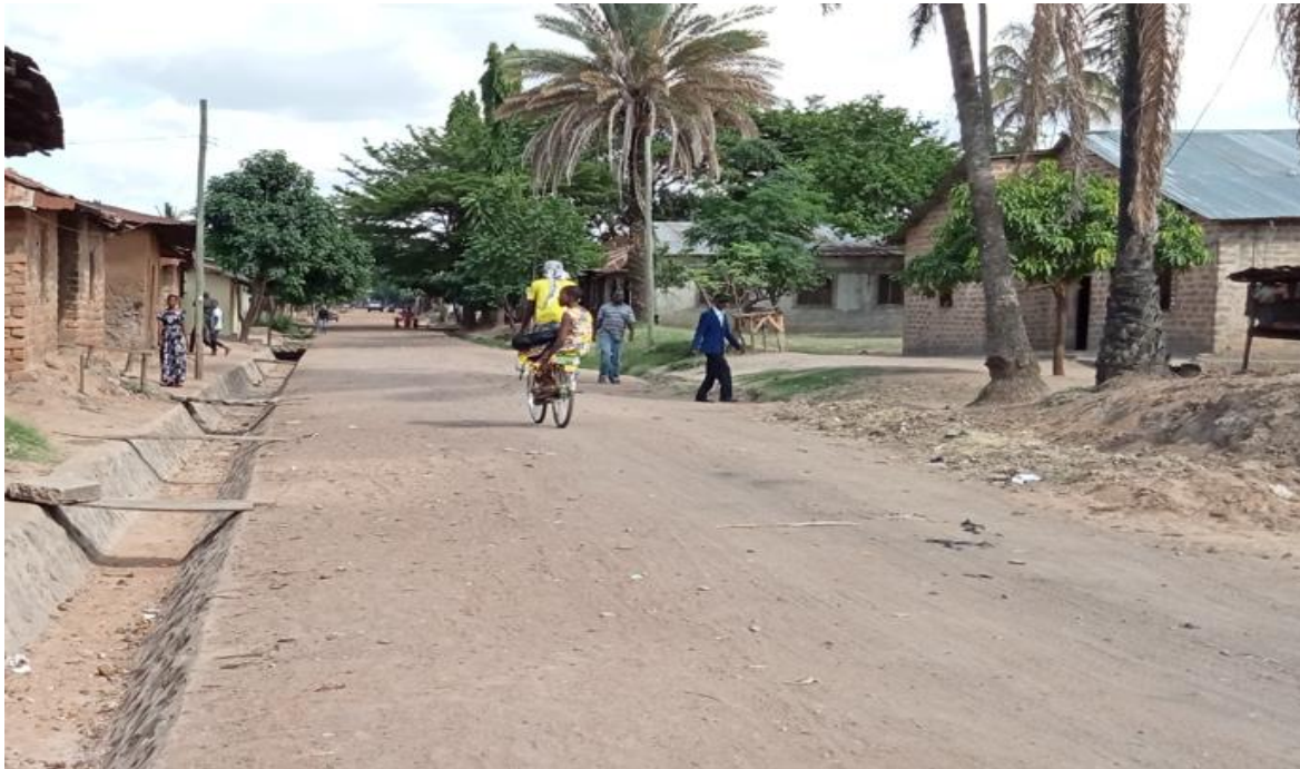
Figure 6.20: Vehicles using the Kanyenye sub-project road
