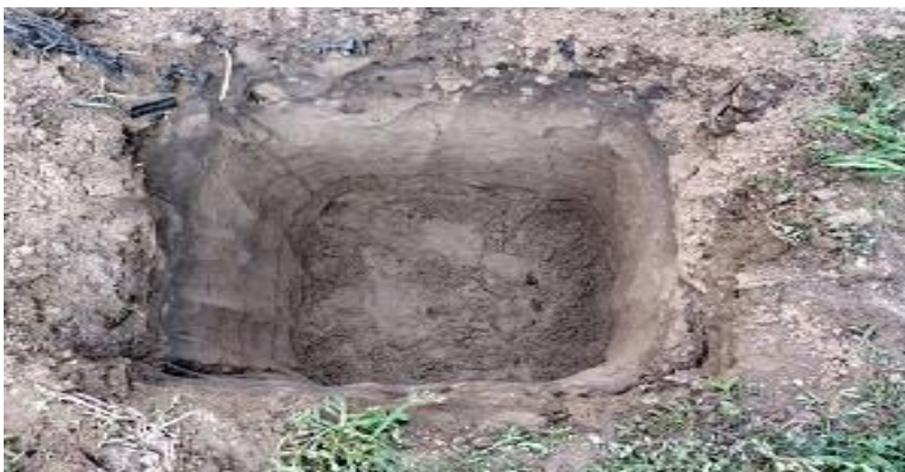
Figure 10: Test pits excavated at km 0+150 (Kanyenye road)
