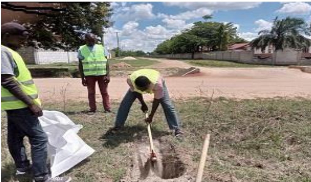
Figure 9: Test pits excavated at km 0+500(Maili tano road)
